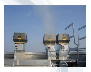
The chimney fan itself is mounted at the top of the flue, on the roof of the tower block, to control the draught in the flue and maintain it at the most fuel-efficient and energy-efficient level possible. Electronic controls sense the fluctuating flow of gases in the flue as the number of boilers firing rises and falls, and control the speed of the fan, and thereby the upward flow of flue gases, appropriately to conditions in the flue.
