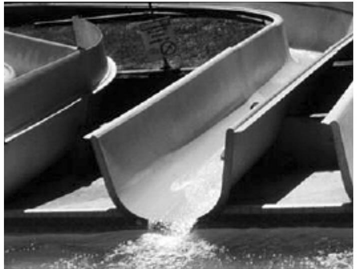
*This slide exit is almost too vertical. A participant coming down head first could hit the concrete bottom.*
